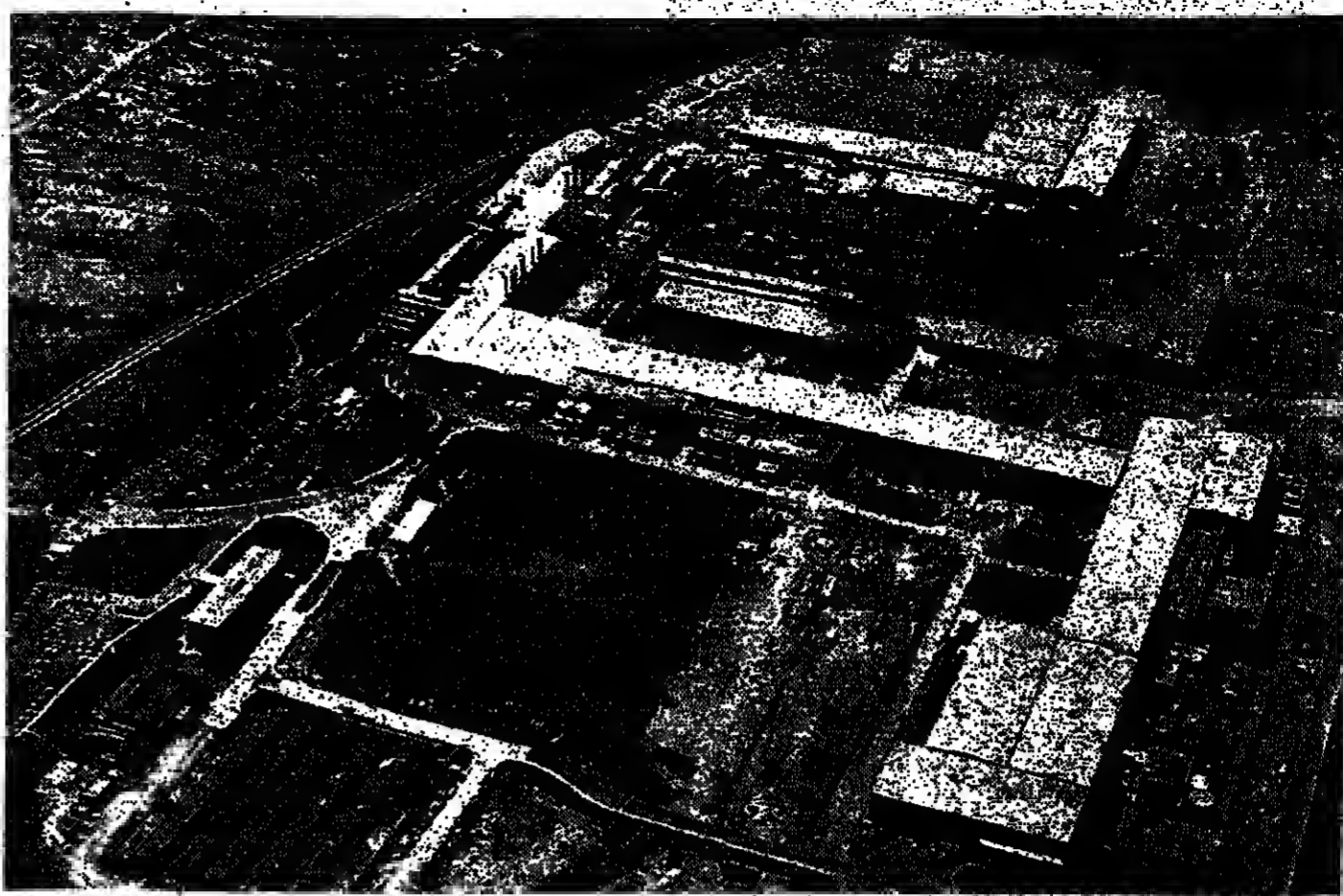
The aluminium roofed buildings house Alcoa's new £35m. rigid container sheet mill at Wainarhydd near Swansea.
